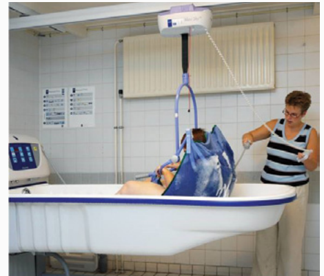
Arjo Ceiling-mounted lift in a bathing room
